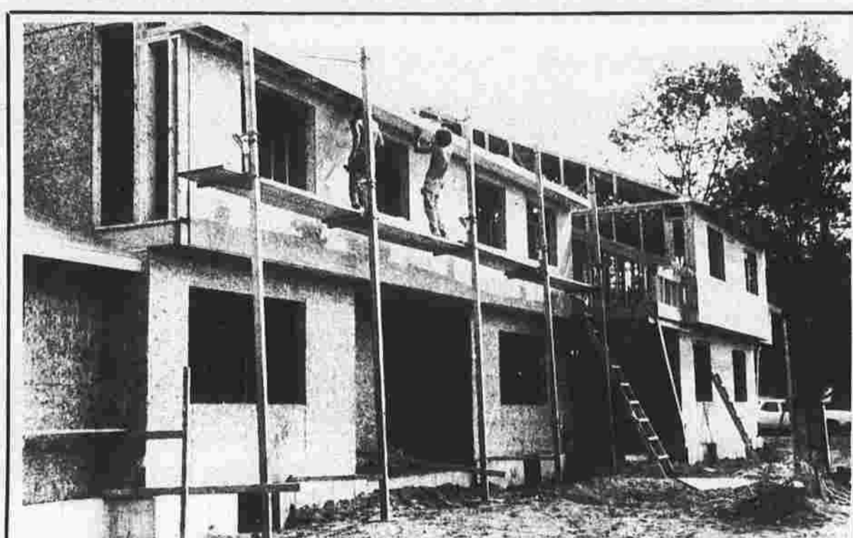
Condo work in progress
